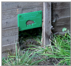
Hedgehog Highway fence gaps provided to allow movement between gardens.
